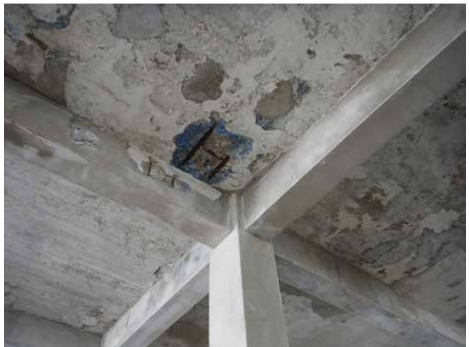
Vertical and overhead repairs prior to using Rapid Set® products.
