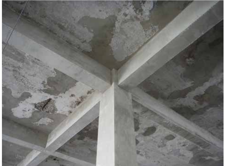
Vertical and overhead repairs after using Rapid Set® products.
