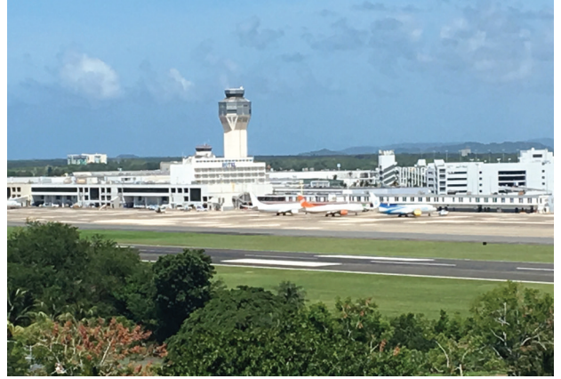
Crews return repaired areas back to service in less than two hours.
